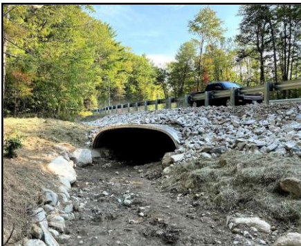
Clover Mill Road Culvert
